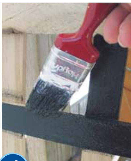
1 APPLY two or three coats of Resene Lumbersider to trellising. When dry, fix to a wall, leaving space behind for ventilation and access.
