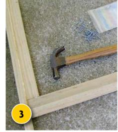
FIX the six vertical struts for the main and side frames into position using PVA glue and nails, and then attach the lower horizontal strut for main frame and side frames. Using the set square, ensure all frames are at 90 degrees.
