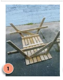
Following manufacturer's instructions, place the tabletop face down on flat ground and fix the leg sections into position, bolting through the underside brackets, as shown.
