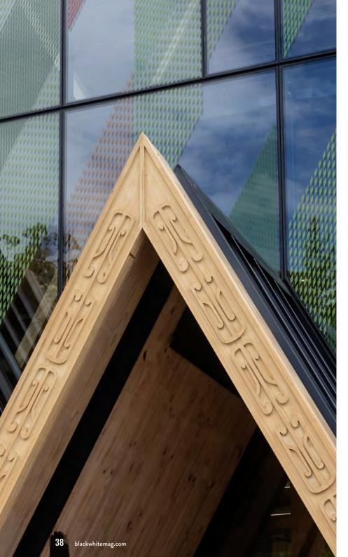
**left and right:** The project team's favourite details include the carved external entrance canopy finished in Wood-X mineral wood oil in Damper – available from Resene ColorShops – and the inventive three-storey engineered timber diagrid, which is clear coated in Resene Aquaclear satin. Exposed steel in Resene Uracryl 404 tinted to Resene Black and exterior fibre cement in Resene Sonyx 101 tinted to Resene Bokara Grey.
