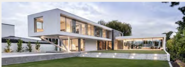
above: This Christchurch home features a Rockcote INTEGRA Lightweight Concrete Facade in Classico acrylic texture finished with Resene X-200 tinted to Resene Half Black White. Design by O'Neil Architecture, www.oneil.co.nz . Build by JTM Construction Ltd. Render cladding by Properly Plastered, www.properlyplastered.co.nz . Image by Stephen Goodenough.
