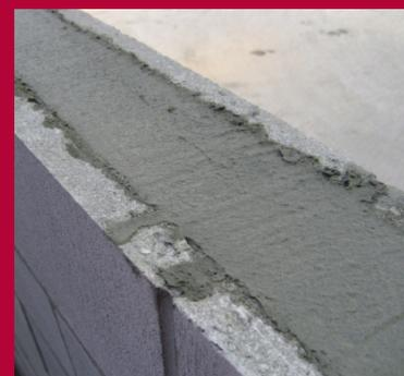
PaintCrete after being levelled off at the top surface of the wall.
