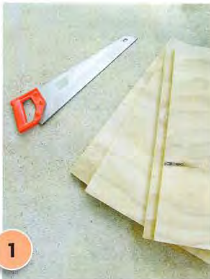
1 Measure and cut the plywood to the dimensions listed above.
