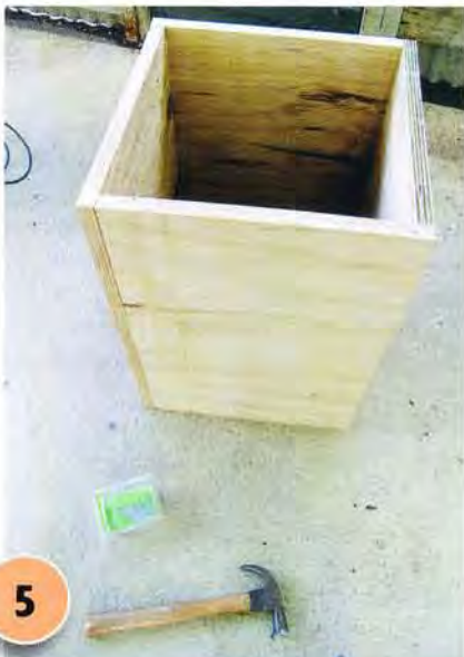
5 Using PVA glue and nails, assemble the four pieces of plywood to create a rectangular structure, as shown. Drill a large hole at the base of one of the sides to accommodate the power cord of the water pump.
