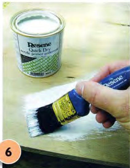
6 Apply one coat of Resene Quick Dry to the plywood structure and allow to dry for one hour.
