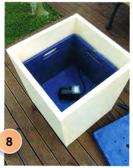
8 Position the water pump as shown – feed its cord through the notch in the crate and hole in the base. Fill the crate with water. Place the drainage tray on top so the pipe and fountain attachment coincide through the central hole. Cover the tray with pebbles.
