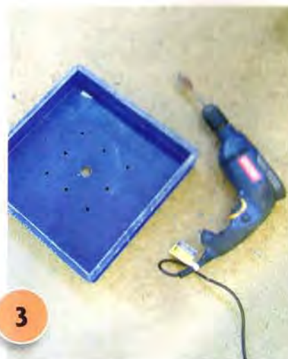
3 Drill eight 10mm drainage holes in the sawn-off base and one larger central hole to accommodate the pump pipe and attachment, as shown.
