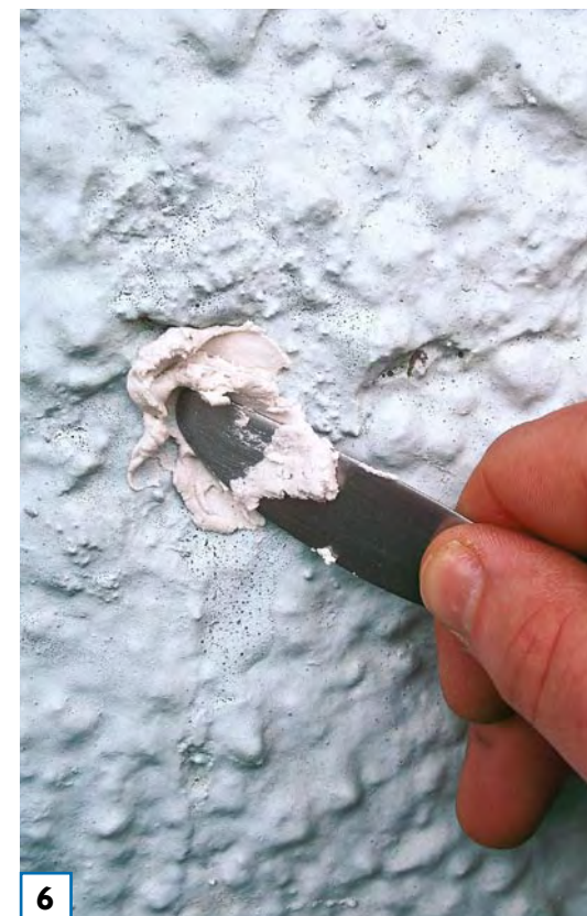
6 Fill any holes in the stucco with exterior masonry filler and allow to dry.
