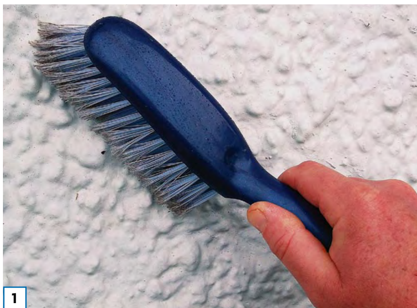
1 Remove any flaking paint or loose stucco with a stiff-bristled brush.
