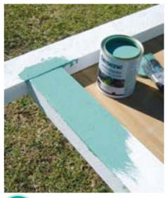
ATTACH the lengths of pine to the top and side edges of the base sheet of plywood with glue and galvanised nails. Paint with two coats of Resene Cutty Sark.
