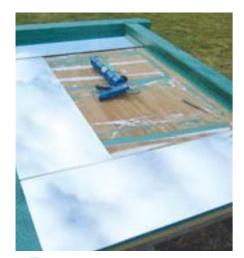
GLUE the mirror panels to the plywood base as shown, sealing around the edges with a bead of silicone sealer. Paint the false gate with two coats of Resene Cutty Sark. Allow to dry overnight.
