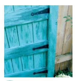
FIX gate in final position with large galvanised nails. Paint hinges on the gate with Resene Nero. Dry brush Resene English Holly and Resene Cutty Sark to suggest woodgrain and highlights.
