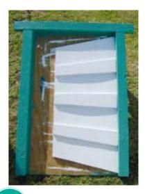
USING the skilsaw, cut the main gate shape as shown with horizontal railings cut from the offcuts of plywood. Prime the edges with Resene Quick Dry Acrylic Primer Undercoat.
