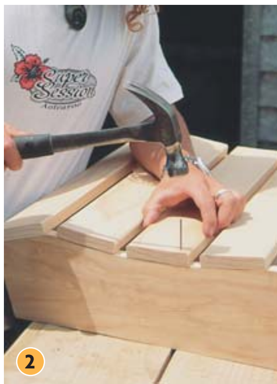
2 Spacing the seat slats 18mm apart, attach slats to base legs using three 50mm galvanised nails at each end of the slats.
