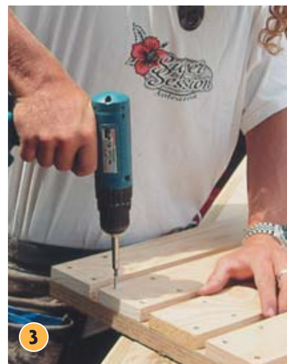
3 To assemble the chair back, lay out five pieces of 100mm x 25mm timber approx 17mm apart and attach to a 100mm x 25mm piece of timber – which will be the base of the chair back. Use four screws for each slat, and ensure the slats are flush.
