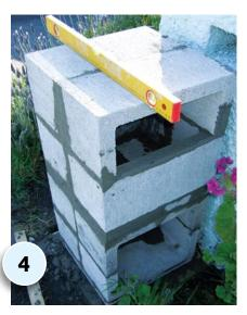
AGAIN, using 10mm mortar joints, lay the 'Standard 200mm Column' on its side (this will form the front mail slot) and the final 'C' type block facing down, as shown. Note: this is a view of the mailbox from the back.
