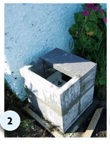
LAY the next two 'C' type blocks, allowing a 10mm mortar joint between each. Use the spirit level to check that the blocks are level in both directions across the top and plumb on each side.
