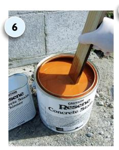
FOLLOWING instructions, mix 1 litre of Resene Concrete Stain Thinnner into the 4 litre can of Resene Concrete Stain in Resene Red Terracotta (Note: this is a two-part mix).
