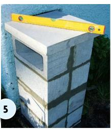
USE a 10mm spread of mortar to fix the 450mm x 450mm paving slab into position, ensuring that it's level in both directions. Leave to dry overnight and remove any excess mortar mix with a wire brush. Leave mortar to cure for 28 days.
