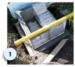
NAIL the pieces of timber to form a square measuring 500mm x 500mm. Dig a shallow hole (approx 10mm deep) measuring 550mm x 550mm. Place the timber frame in the hole, ensuring that it's level. Mix up some concrete and trowel this into the frame, levelling off with an off-cut of wood. Place two capping blocks on top of the wet concrete base. Mix up some builders' mortar mix and lay the first two 'C' type blocks on top, as shown.
