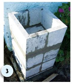
LAY another two capping blocks with mortar joints of 10mm and two more 'C' type blocks, as shown. Continue to use the spirit level to check top is level and sides are plumb.
