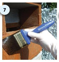
USING the 75mm brush, apply one coat of Resene Red Terracotta to the mailbox and final two 'Plain End Half High' blocks - take care to ensure even coverage. Allow to dry for 4 hours and apply a second coat. Once dry, place the two blocks on top of the mailbox to form small planters - note: to ensure good drainage, do not mortar these into position.
