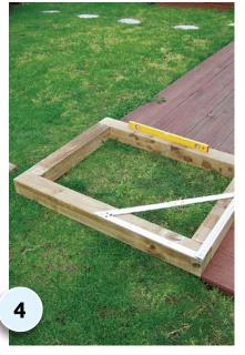
Place this first frame into position – using a spirit level and large setsquare to make sure it's level and square.
