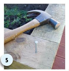
Repeat step three to make a second frame and fix this to the first frame, with agenerous amount of construction glue and a nail at each corner. (Drill a pilot hole first). Repeat this until you have five frames in position. Leave overnight for glue to dry.
