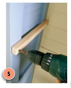
Measure and cut six lengths of 25mm battening to form the shelf supports. Fix to the inside of both side walls of the unit with PVA glue and screws. Measure and cut three piece of plywood to form the shelves.
