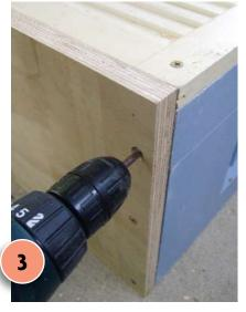
Measure and cut a piece of plywood to form the base and fix into position with PVA glue and screws. Measure and cut a piece of plywood to form the roof.
