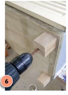
Measure and cut four 50mm lengths of 50mm timber and fix to the base of the toolshed with PVA glue and screws to form the feet.
