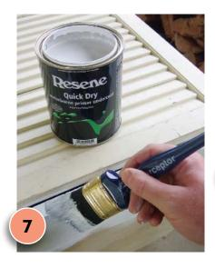
Lightly sand the cupboard doors. Sand and spot prime with Resene Quick Dry any bare wood where old paint has chipped. Prime all the sides of the plywood with Resene Quick Dry. Allow to dry for two hours.
