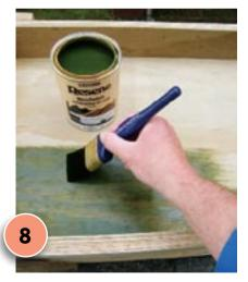
Stir the Resene Woodsman penetrating oil stain with a wide, flat paint stirrer. Apply two coats to the unit (brush in the direction of the grain). Leave each coat 24 hours to dry. Slot the sink in place.
