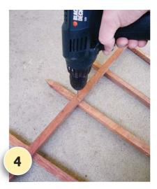
Drill pilot holes, as shown, and fix with PVA glue and galvanised clouts.
