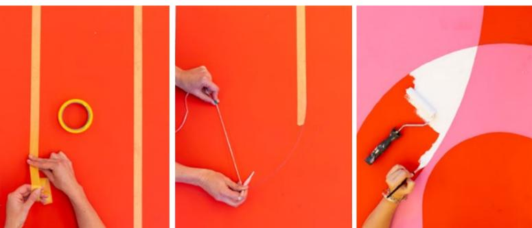
**Step 1:** Using the above method, draw a 104cm radius circle in the centre of the wall. Placing the centre point 30cm up from the floor. From the left wall measure 37cm in and 145cm up from the floor and masking tape on the left side from point to point. Repeat this step 64cm in from the left and 145 cm up from the floor and masking tape on the right side from point to point.
