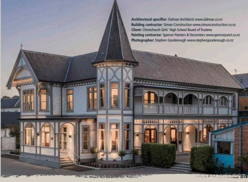
A series of steel portal frames on the ground floor were installed to replace walls that were removed and provide additional seismic strength. All existing lathe and plaster linings (which were severely damaged) were removed and replaced with plywood bracing and plasterboard bracing linings. The foundations were also significantly strengthened.
