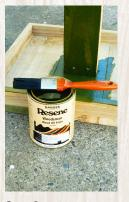
**Step 8** Apply two coats of Resene Woodsman tinted to Resene Grey Green to the feeding table, allowing the first coat to dry before applying the second.
