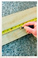
**Step 1** Measure and mark three 450mm lengths of fence paling.
