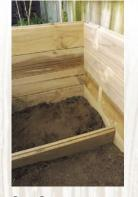
Step 3 Build up the sides of the deck, as shown, using the remaining 1800mm lengths and 1000mm lengths of tongue and groove landscaping timber. Again, fix with 100mm screws.
