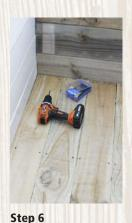
Lay the fence palings in position and fix with 65mm screws. Measure, mark and cut the final fence paling to fit.
