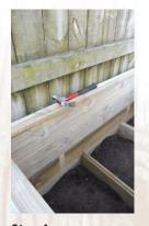
Step 4 Measure, mark and cut the fence capping to fit along the sides of the deck and fix into position with decking nails.
