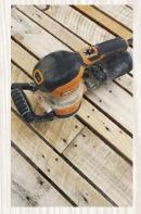
Step 6 Sand the entire table using the electric sander and then wipe off any sanding residue with a clean cloth.
