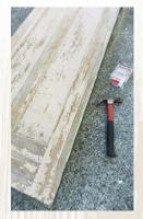
**Step 2** Attach the wooden door to the underside base, fixing with 65mm nails.
