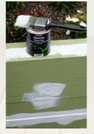
**Step five** Spot prime any filled gaps and areas of bare wood with Resene Quick Dry. Allow two hours to dry.
