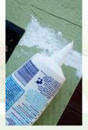
**Step four** Fill any holes or gaps in the wood with exterior filler and allow to dry. It's easy to freshen up a previously painted wooden raised bed with a little bit of help from Resene.
